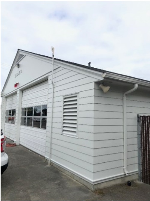
New Paint at Station 3!
